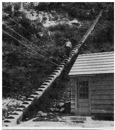
The swinging bridge at Verlot provided access to the Mt. Pilchuck trail, and was built with the cooperation of the Forest Service, CCC, and a couple of well-known Silverton locals . . . the Shedin brothers! The CCC cut the huge tree from which steps were hewn, to be used as a stairway near the powerhouse of the Verlot Ranger Station. There was no limit to the projects undertaken by the intrepid young men of the CCC.
